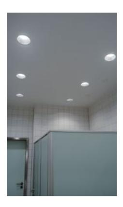
All glass inserts provide splash water protection. Luminaires with permanently glued-in glass covers attain protection mode IP43 (from below) when installed in closed ceiling systems.
